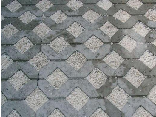
Plate 4-32 Example of filter drains and permeable surfaces
